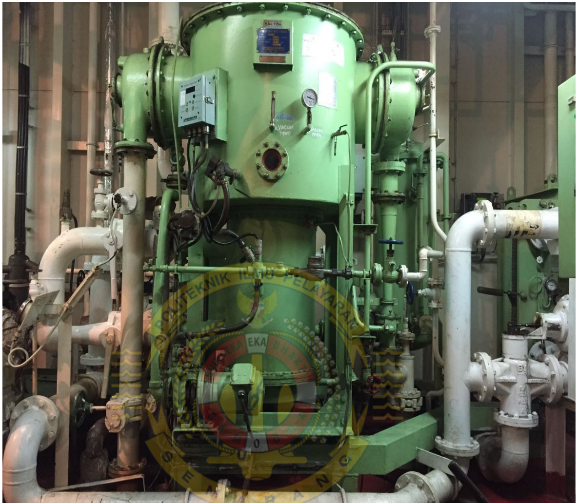
Gambar Fresh Water Generator SASAKURA Type KM 25 Sumber: Dokumen Pribadi 2016
