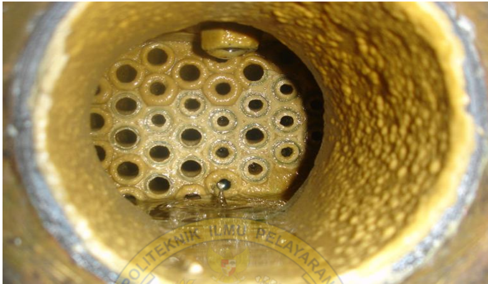
Gambar Tube Side Kondensor MV. Kartini Samudra
