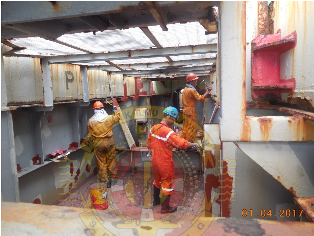
Perawatan Cross Deck
