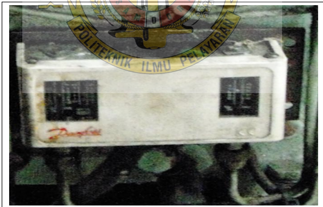
Gambar 8. High and Low Pressure Control.
