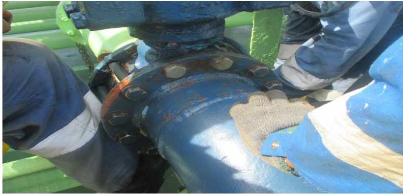
Gambar 1. Proses pembongkaran valve cargo no.2
