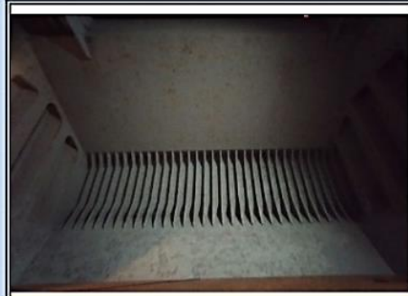
4. Stbd side shell and tank top
