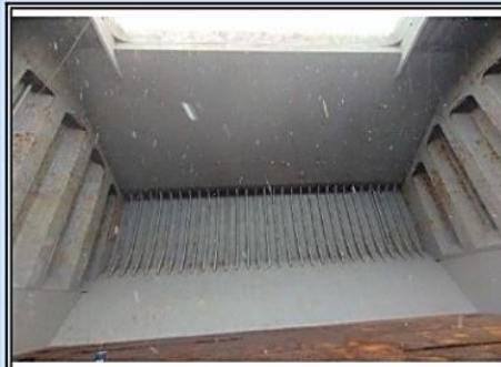
4. Stbd side shell and tank top
