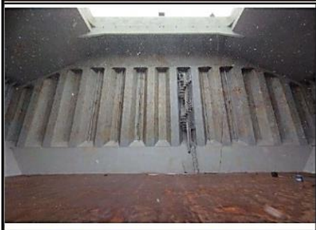
1. Forward Transverse bulkhead
