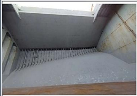
4. Stbd side shell and tank top
