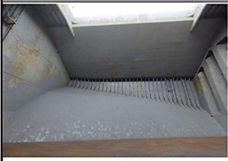
3. Port side shell and tank top
