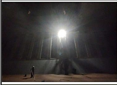
1. Forward Transverse bulkhead
