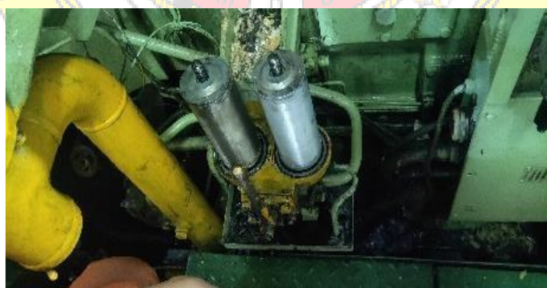
Gambar filter L.O main engine
