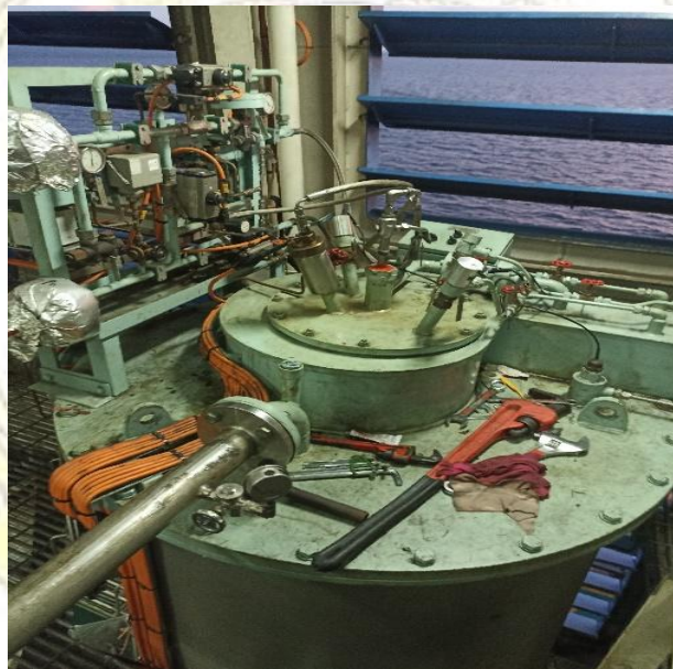
Gambar 4. 22. Inert Gas Generator MT. Panderman
