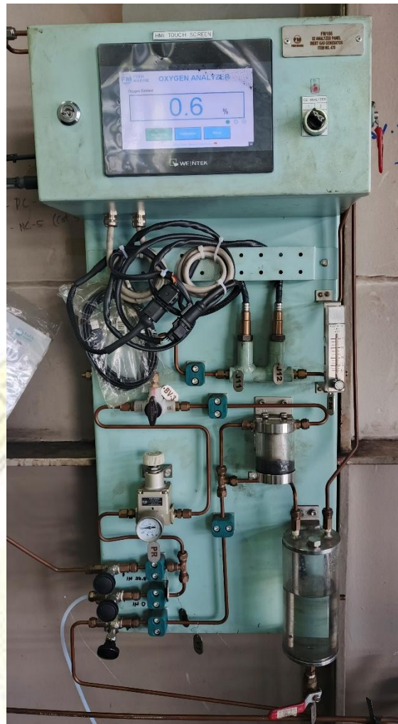
Gambar 2. 14. Oxygen Analyzer
