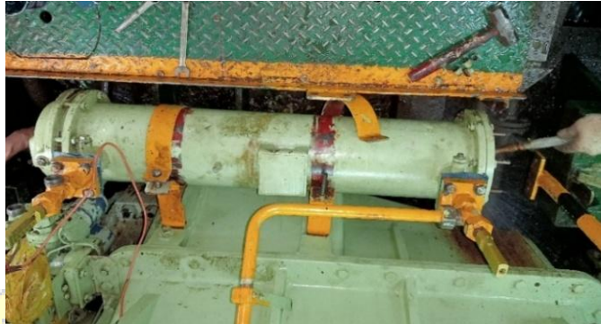
Gambar 2. 3 Lo Cooler Shell and Tube
