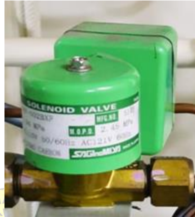
Gambar 2.7 Solenoid valves
