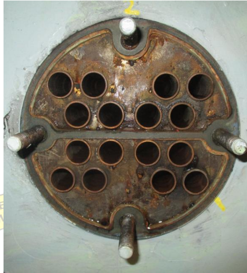
Gambar 2.3 Water cooled condensers type shell and tube
