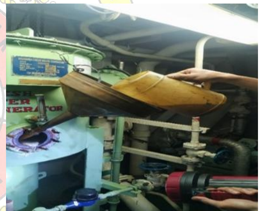
Gambar 15. Pemberian chemical melalui sight glass
