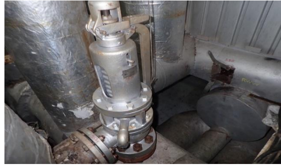
Gambar 2.6 Safety valve Sumber: Dokumentasi Peneliti 2023
