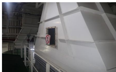
Gambar 2.12 Steam air heater Sumber: Dokumentasi Peneliti 2023
