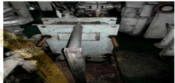
Gambar: 4.1 *Fresh water cooler* di kapal MT. Iris
