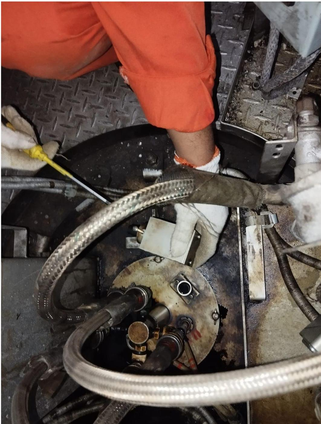
**LAMPIRAN 9 Automizer Main Burner Auxiliary Boiler**
