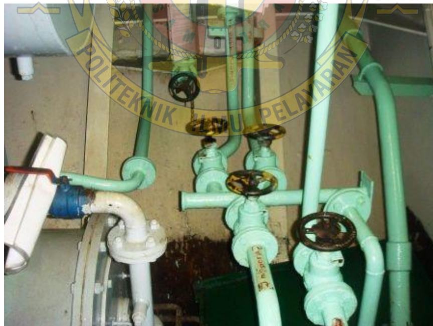
Gambar. 2 diagram piping oily water separator.
