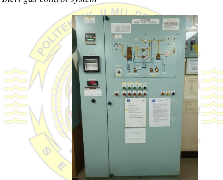
Gambar 2.7 ( inert gas control system MT. Luna Erawan)
