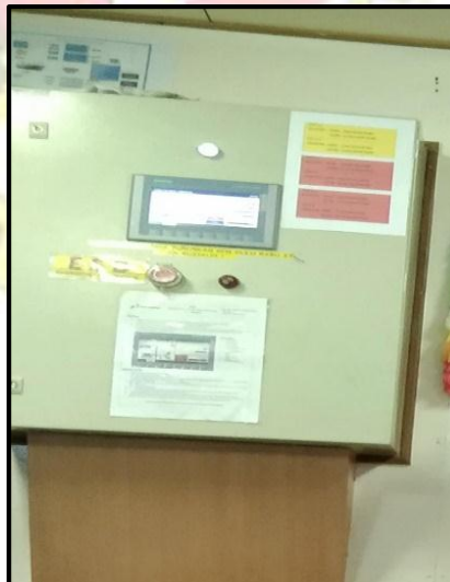
Gambar 2. 12 ESDV ( Emergency Shut Down Valve ) Sumber : Dokumen Pribadi
