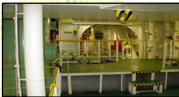
Gambar : 2. 10 Pump Room
