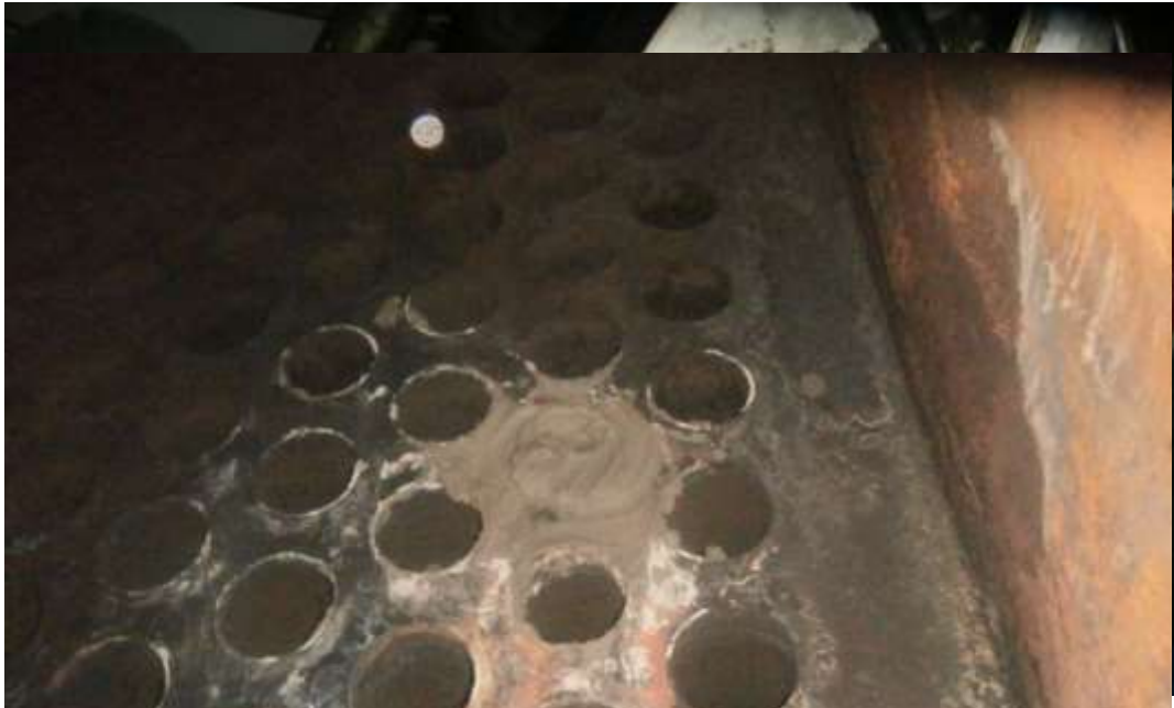
Lampiran 1 proses plugging economizer tube
