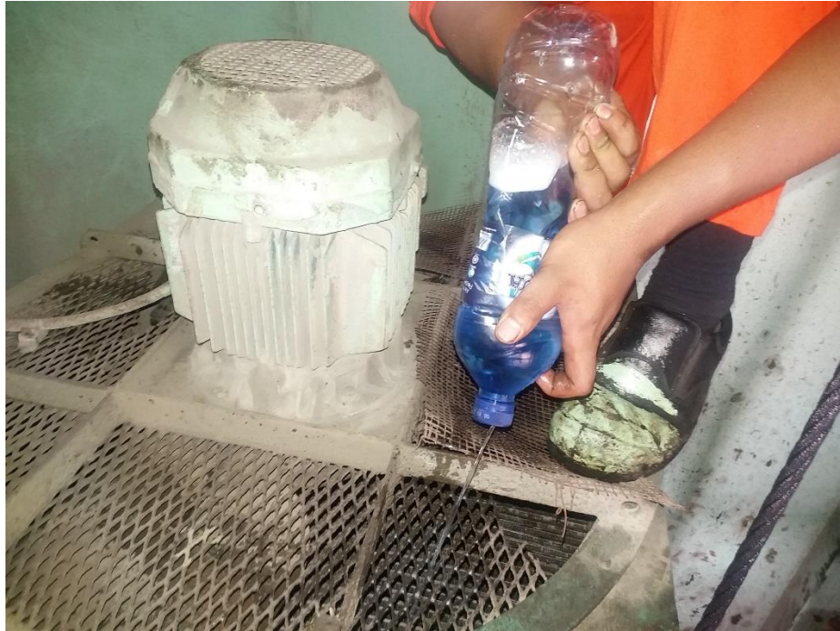
Gambar: Cleaning Oil Cooler
