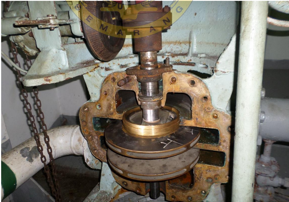
Gambar 14 Pembongkaran Emergency Fire Pump
