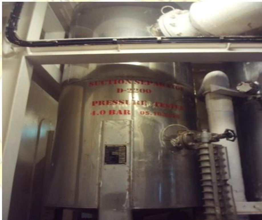
Gambar 2.1 *Knockout Drum*
