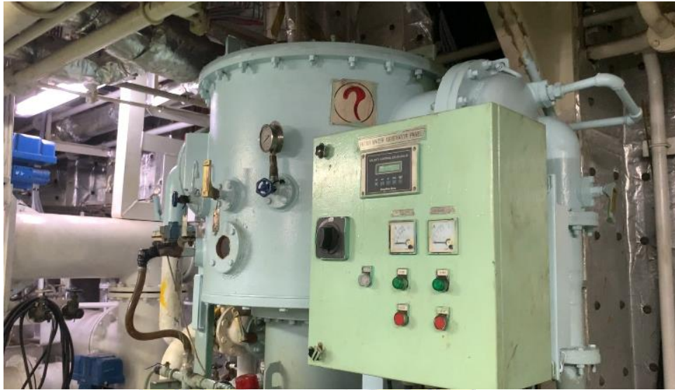
Gambar 2.1 Fresh Water Generator
