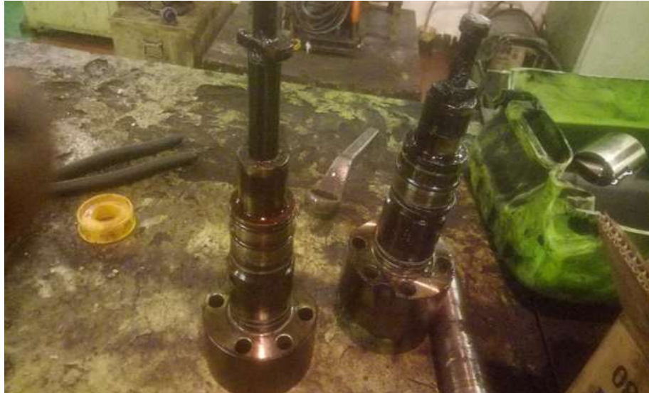
Macetnya Plunger Barel Fuel injection pump Generator
