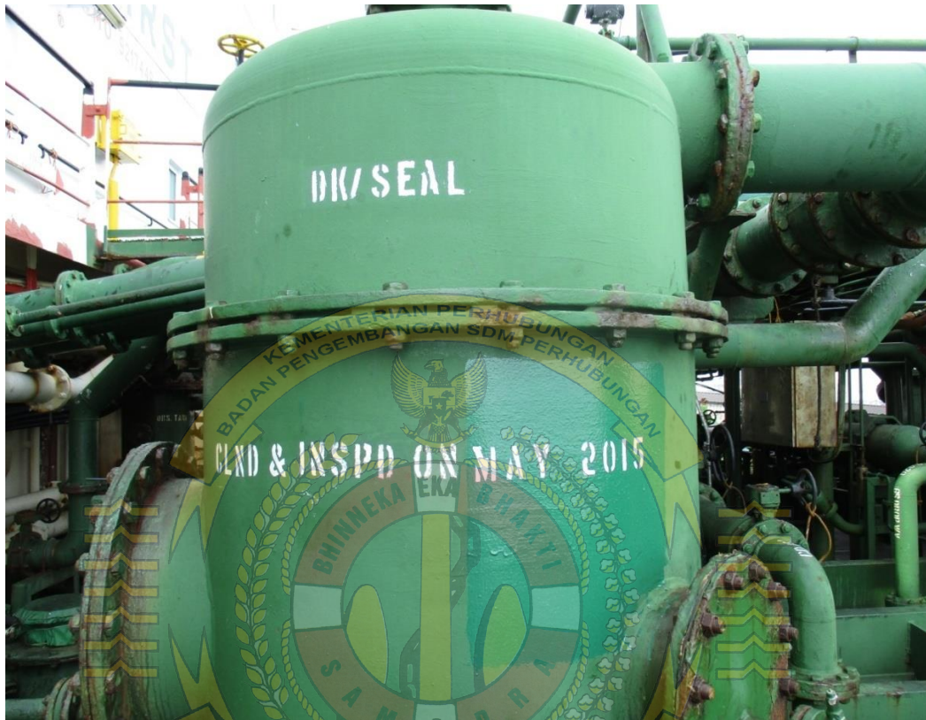
Gambar 1 Deck Water Seal
