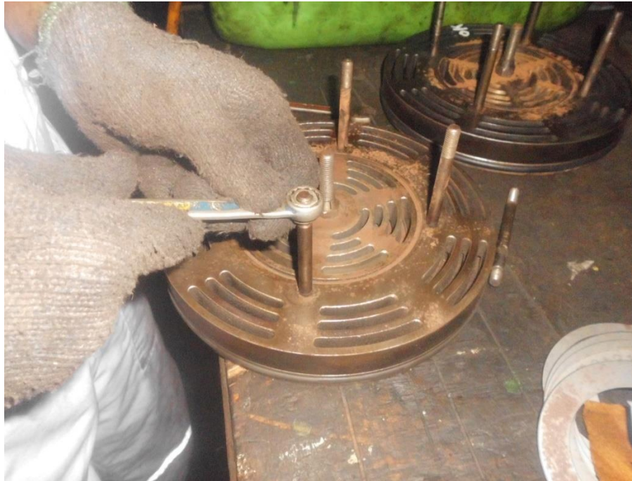
Gambar Kondisi Pengecekan First Stage Valve
