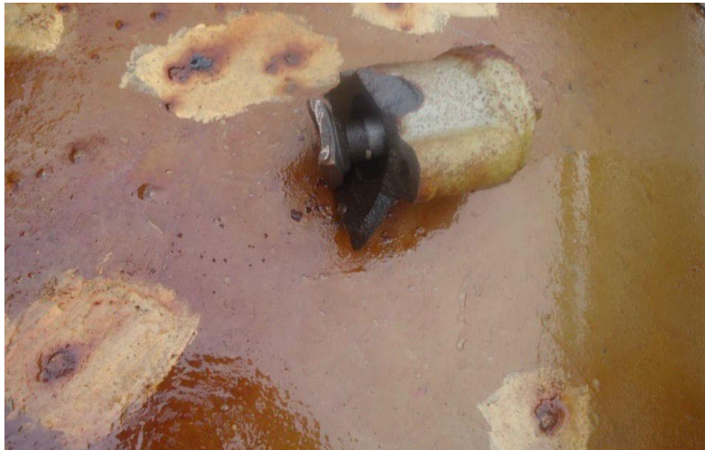
Lampiran 6 kondisi Hydraulic oil pump pecah
