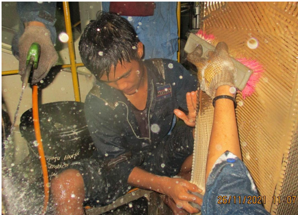
Proses pembersihan fresh water cooler
