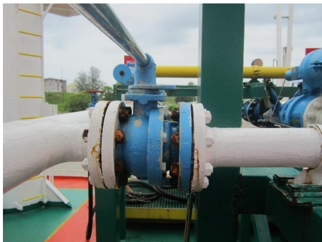
Gambar : Line Crossover Cargo Compressor
