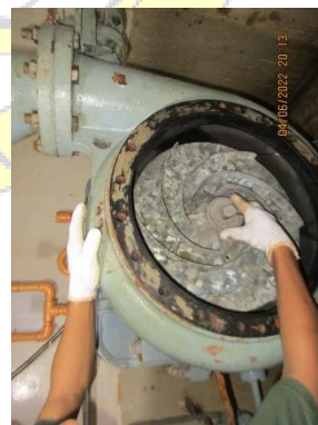
Pemasangan Mechanical seal
