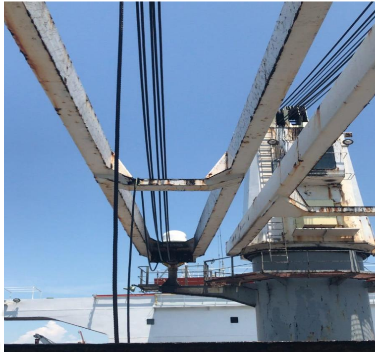
Proses penggantian wire crane
