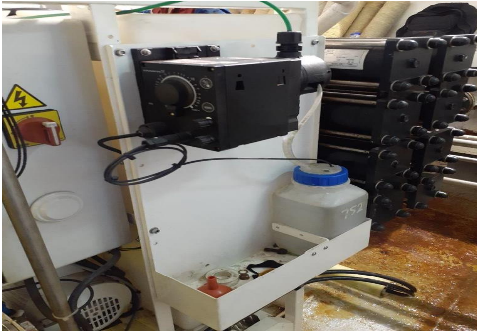
Gambar 10 : Antiscalant Dosing Pump
