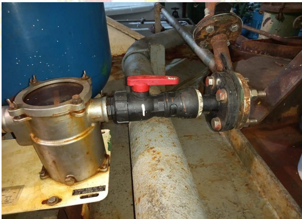
Gambar 11 : Filter Strainer
