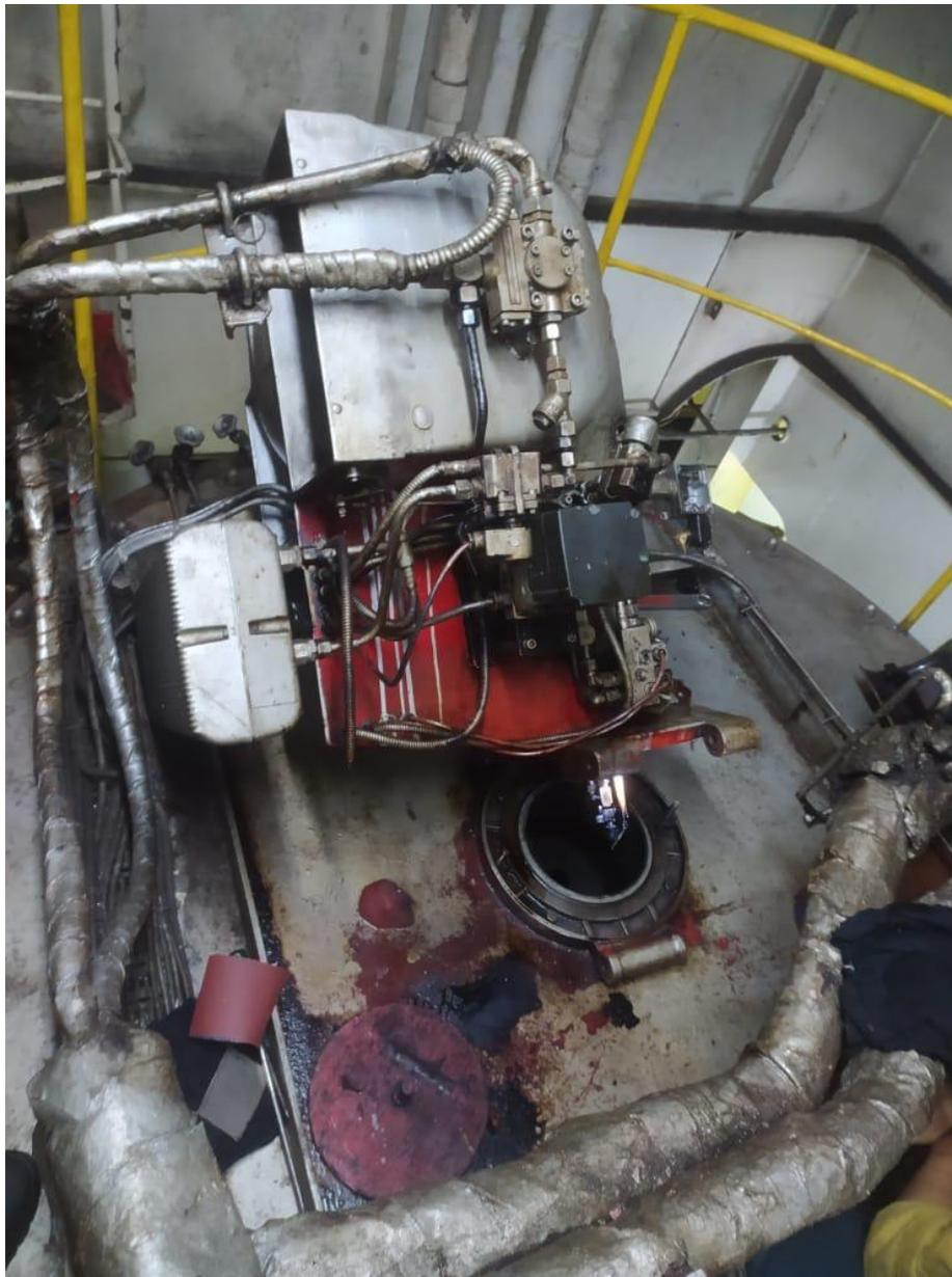
Gambar Overhaul *Burner Thermal Oil Heater*
