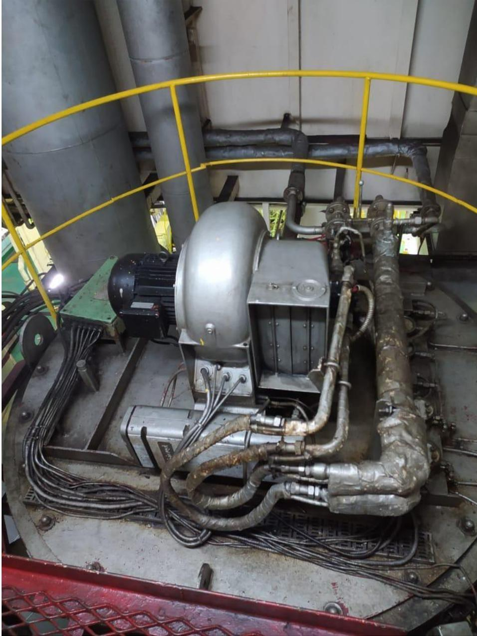
Gambar *Burner Thermal oil heater*
