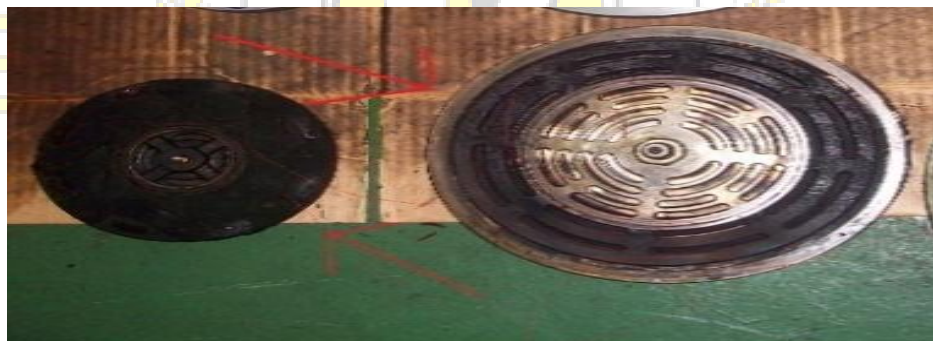
Pembersihan Low Pressure Valve Main Air compressor
