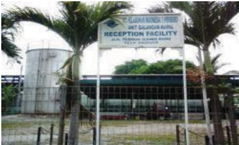
Figure 11. Waste collection and disposal facilities.
