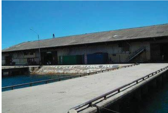
Figure 3. Warehouse line I.
