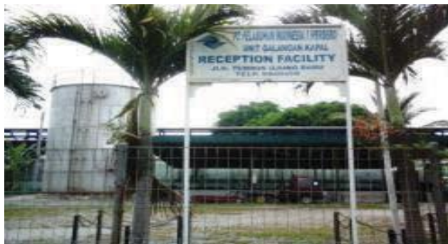
Figure 12. Waste collection and disposal facilities.
