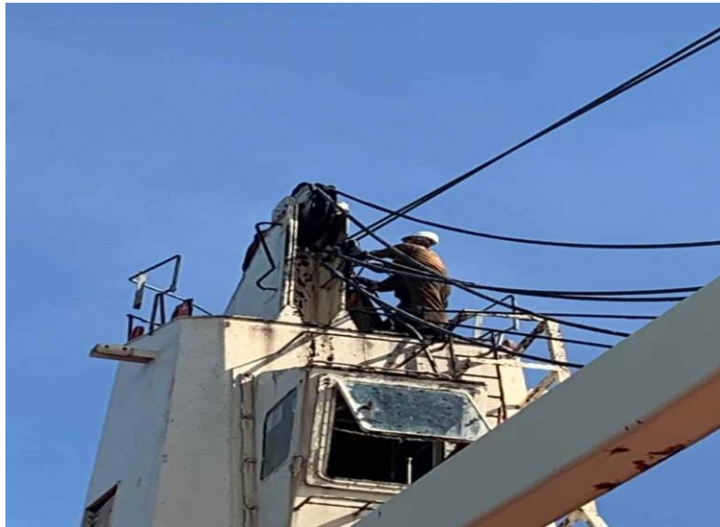
Lampiran 3.3 Kegiatan Penggantian Wire Luffing Crane
