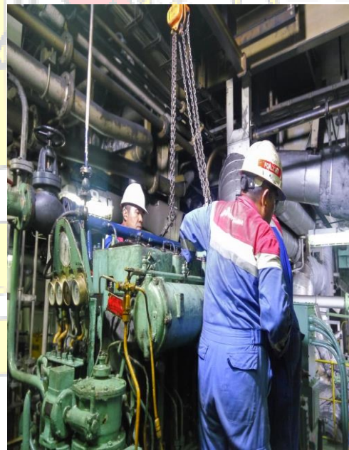
Kegiatan overhaul diesel generator
