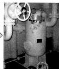
Open drain valve for knock-out drum
