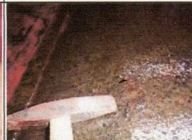
Close up section of tank top – Wet Condition. When dry became yellow.
