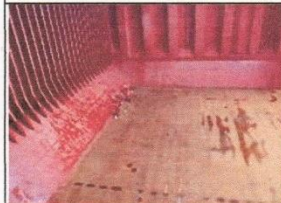
Example: Tank Top No.4 Hold.
