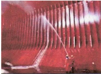
Thoroughly washed down side frames in Hold by S.W.
