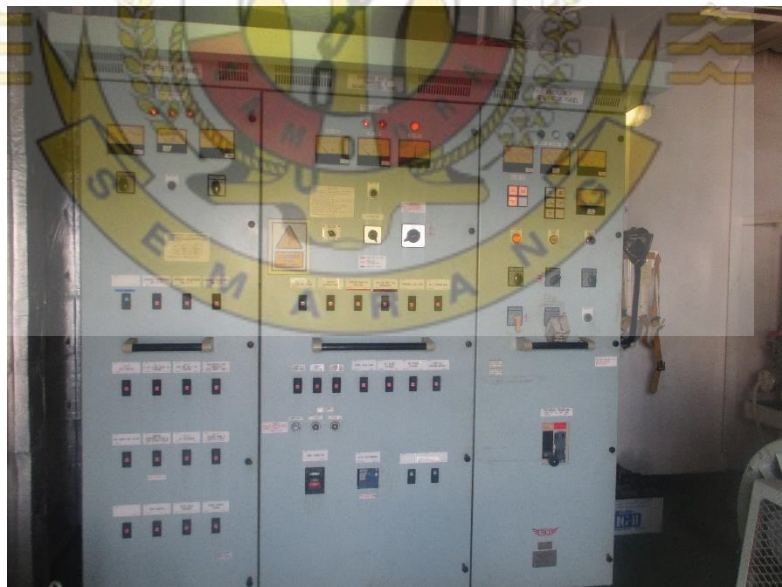
Main Switch Board Emergency Generator
