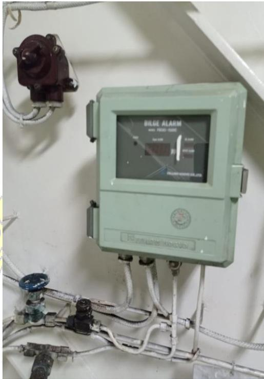
**Gambar 15 ppm alarm bilge (Oil Content Meter)**
