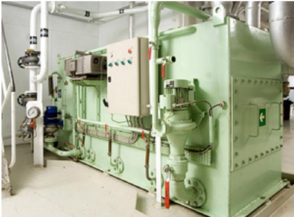
Sewage Treatment Plant
