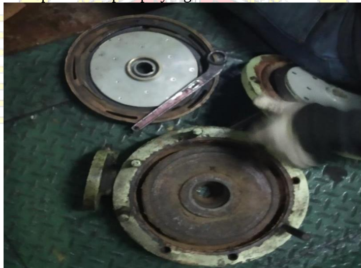
Penggantian impeller feed water pump
