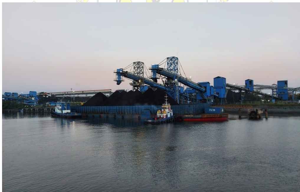
Tanah Merah Coal Terminal (TMCT)
