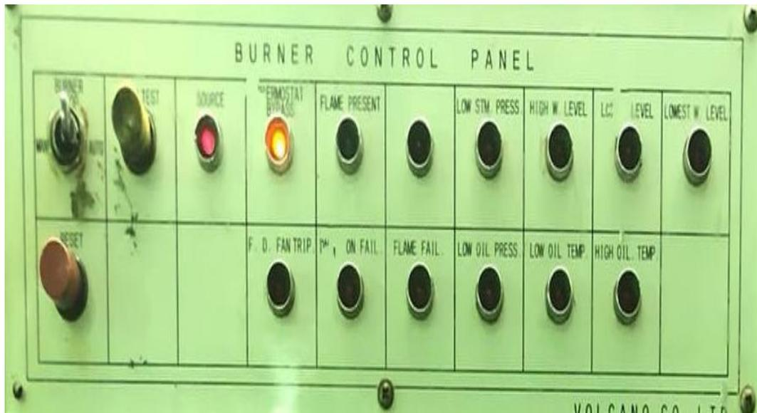
**Gambar Burner Control Panel Auxiliary Boiler**
