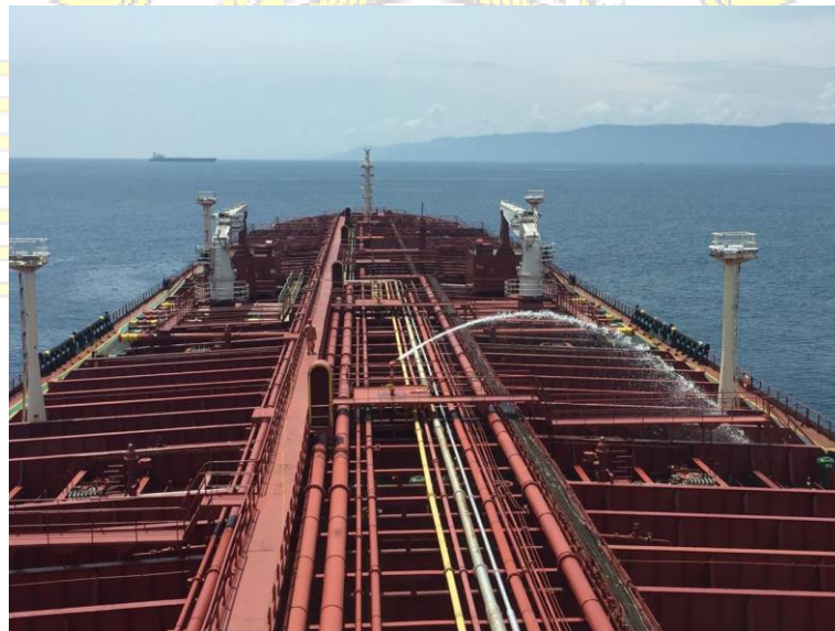
Pelaksanaan tes fix fire extinguisher (foam system)
