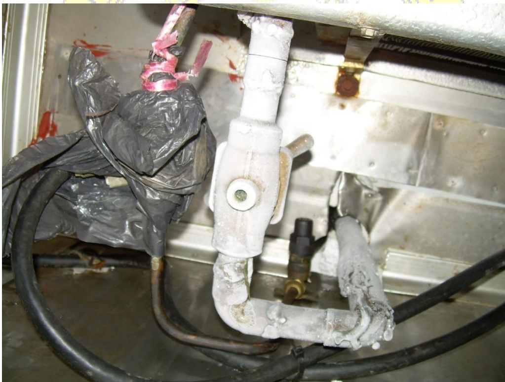
Gambar 2.3 Expansion Valve
