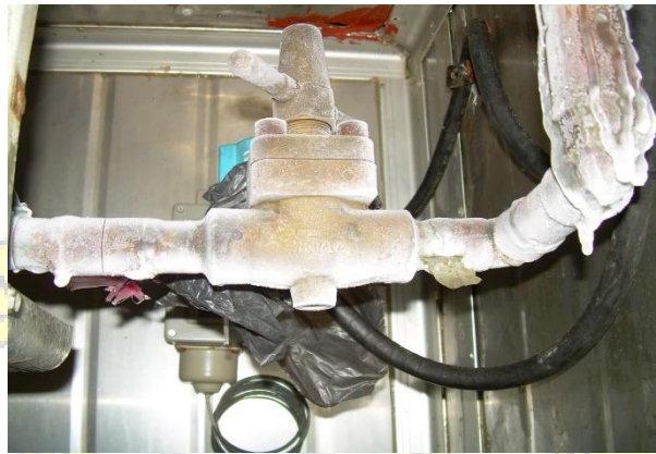
Gambar 2.3 Expansion valve
