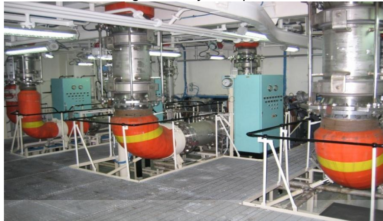
Ruang Low Duty Heater
