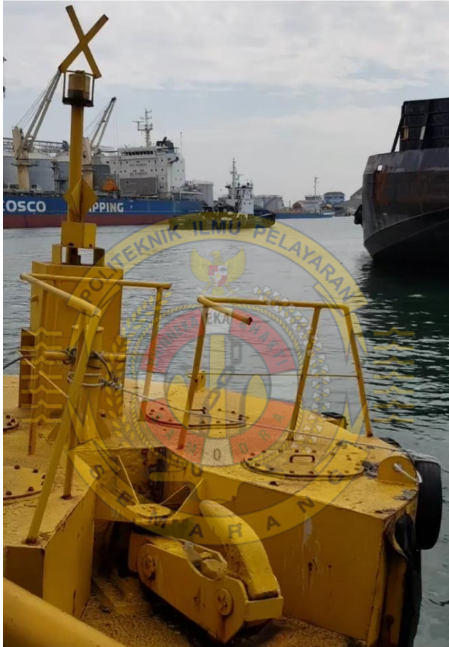
Single Bouy Mooring
