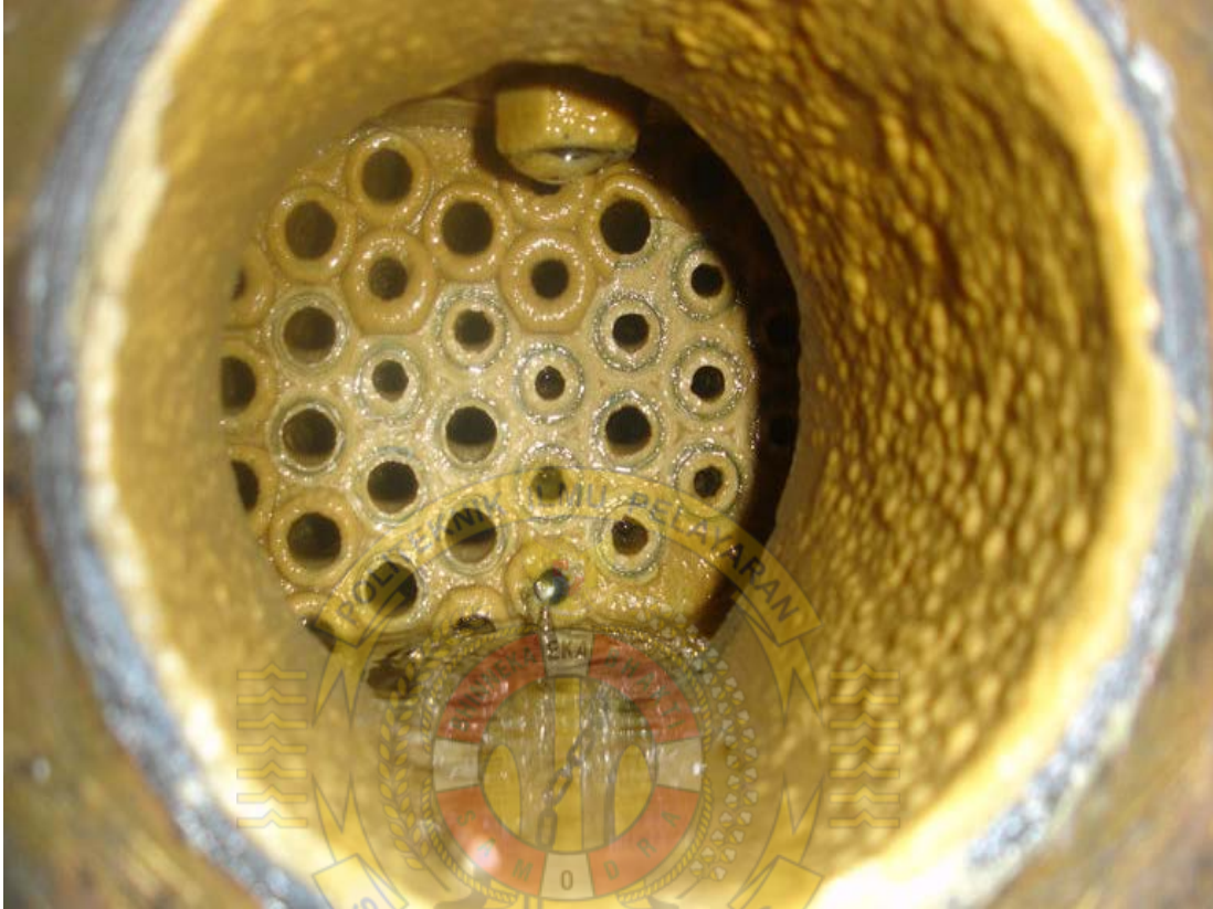
Gambar Tube Side Kondensor MV. Oriental Galaxy
